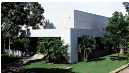
PLANT - I Mannur, Chennai
